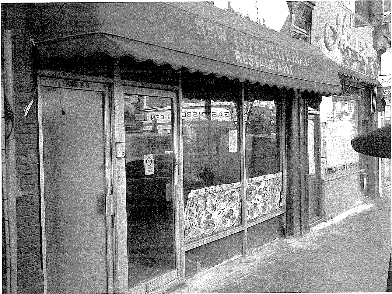
Front of premises on green lanes N4
